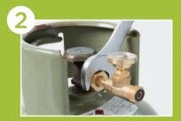
Tighten the GasStop using the correct tool.
